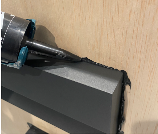
Fig.5: Apply silicone around exterior perimeter.
