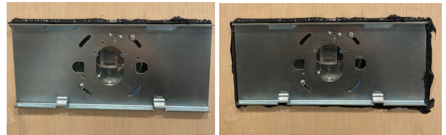
Fig.3: Apply Silicone around mounting bracket.
