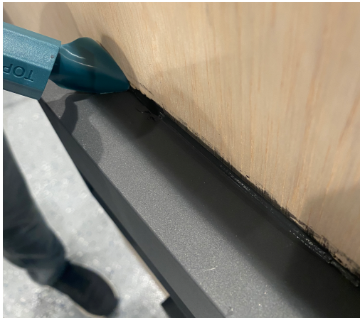
Fig.6: Create a clean finish and remove excess silicone.
