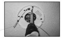
(3) Secure suspension cable loop around the hook inside the top of the fan body.
