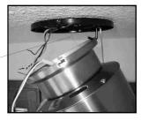
With fan safely suspended by hook, make wire connections with wire nuts included in fan hardware package as described in the control installation instructions. If using the optional #003 or #004 control, the receiving unit should be connected at this time and placed inside the canopy.
