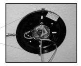
**(6)** Lift fan body and hang from ceiling plate hook. The hook should go through one of the closed holes in the canopy.
