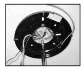
(5) Remove two of the set screws from the ceiling plate opposite one another and set aside for step (7). Loosen the other two without removing them from the plate.
