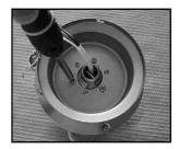
**(4)** Using the existing screws from your junction box, or the machine screws from the fan hardware package, secure the ceiling plate to ceiling junction box. The electrical wires must be accessible through the hole in the center of the ceiling plate.
