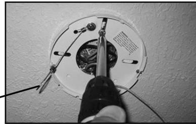
**(9)** Secure suspension cable loop around the hook inside the top of the fan body.
