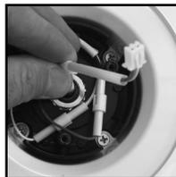
Join ends of bridge connector wires with wire leads from fan. Position wires so that connectors are flat and to side of three posts inside connection cavity.
