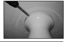
(12) Install bottom cap if your fan does not have a light kit or the glass diffuser if your fan does have a light kit. In either case, rotate clockwise until cap or diffuser comes to a stop.
