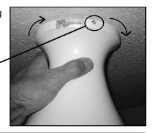
(8) Insert and firmly tighten three set screws. Hintdo not tighten down set screws until all three are partly screwed in.
