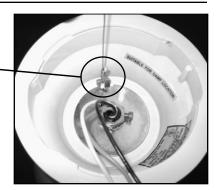
(7) Lift fan body and carefully align collar with ceiling plate. Tabs on ceiling plate should seat into channel on inside of fan collar. Rotate fan so that set screw holes on fan body align with set screw holes on ceiling plate.
