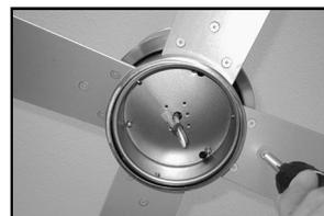
**(11)** Attach bottom cap to fan body by aligning slots on cap with fittings inside fan body, and rotating clockwise, or proceed to step **(12)** if you are using the optional light kit.
