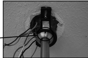
With fan safely suspended by bracket, make wire connections with wire nuts included in hardware package as described in the control installation instructions. If using the optional #003, #004 or #005 control, the receiving unit should be placed inside the arms of the hanging bracket and connected at this time.
