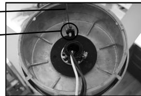
(6) With fan safely suspended by cable, make wire connections with wire nuts included in hardware package as described in the **Control Installation Instructions**. If using optional #003, #004 or #005 controls, the receiving unit should be placed inside the top of the fan and connected at this time.
