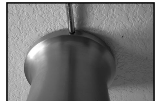
Secure with set screws
