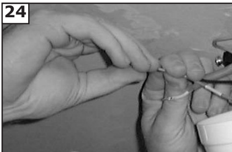
24 Make wire connections to power source using wire nuts provided. Make sure that no filaments are outside of the wirenut. After making the wire connections, the wires should be spread apart with the grounded conductor and the equipment-grounding conductor on one side of the outlet box and ungrounded conductor on the other side of the outlet box.
